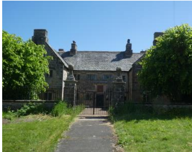
Newby Hall, north elevation
